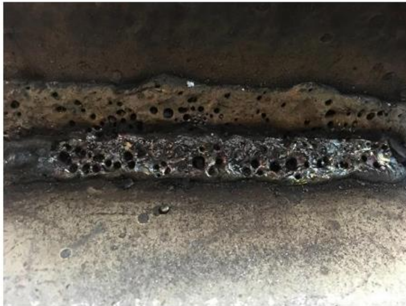
Welding porosity: an example of a quality related issue.
